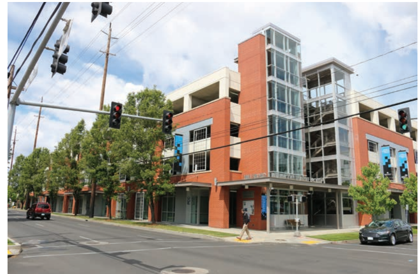
Hillsboro Center is currently located within the Hillsboro Intermodal Transit Facility.
