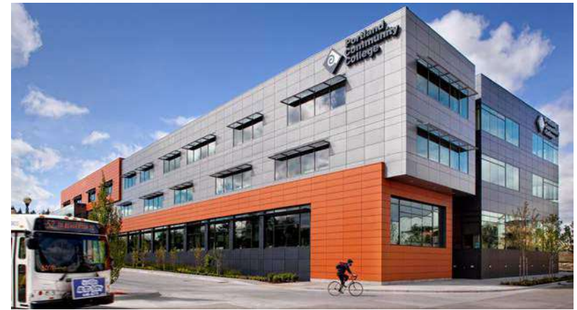
Willow Creek Center
