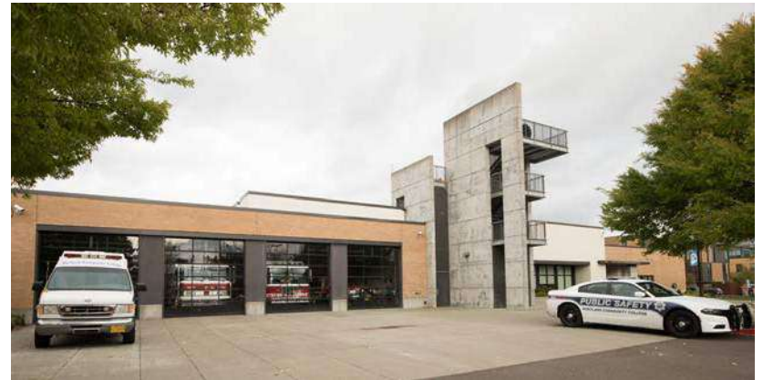
With roll-up bays for Fire Protection Technology program vehicles, the program often utilizes parking lot 5 to the south of the building for training exercises and other activities.
