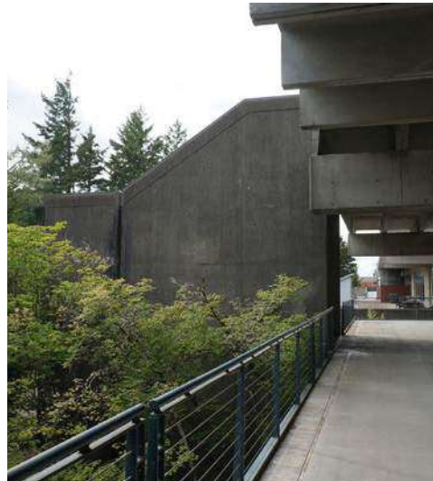
Existing concrete stair tower west of SS
