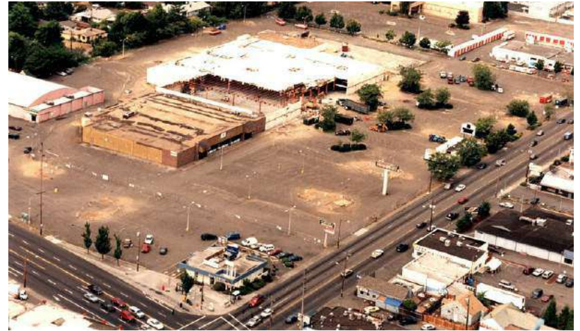
Southeast Campus being retrofitted from a shopping center (early 2000s)
