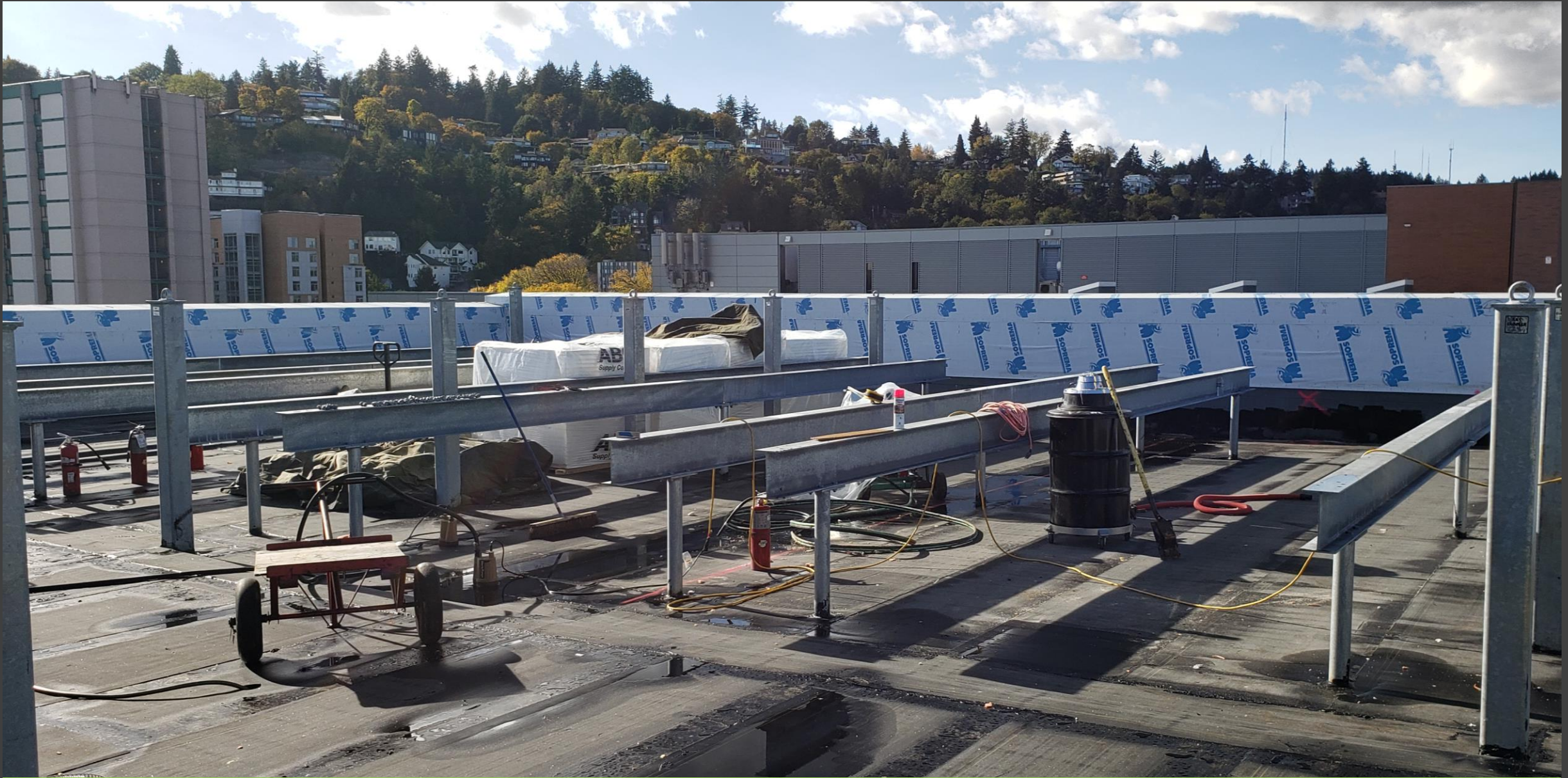
Roof – Solar Panel Supports
