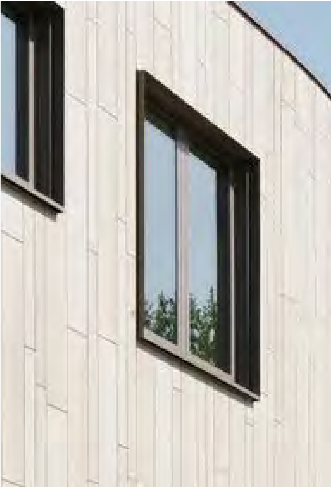
Assembly principle: screws on aluminium substructure
