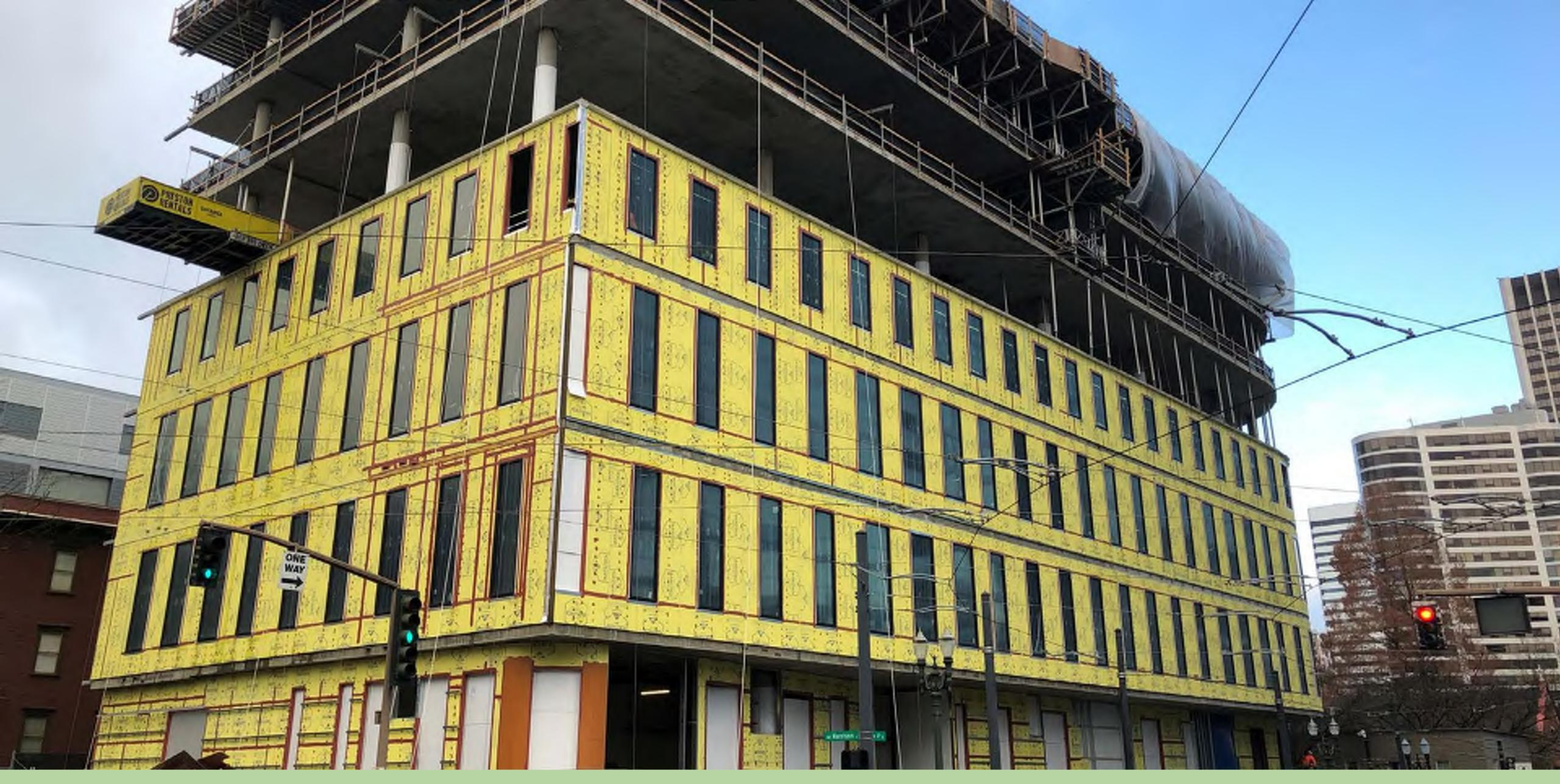
• Weather barrier being installed at slab edge.
