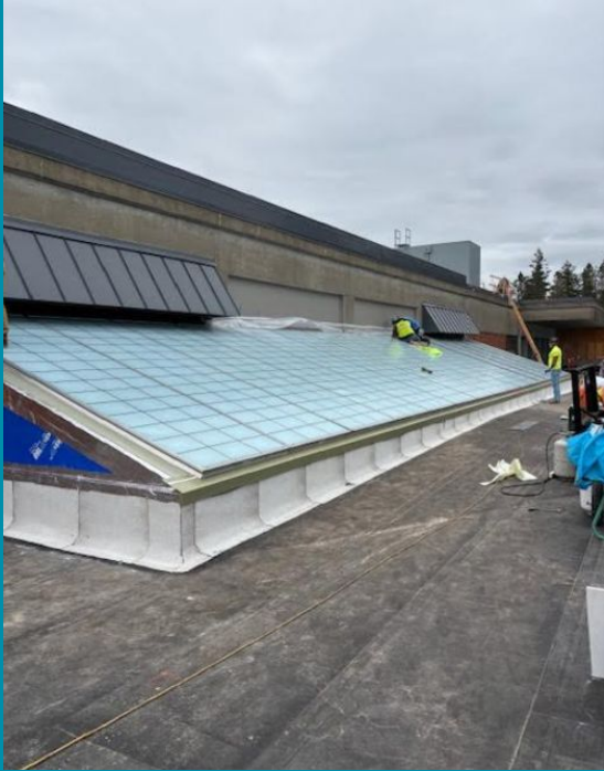
Skylight install and new roof
