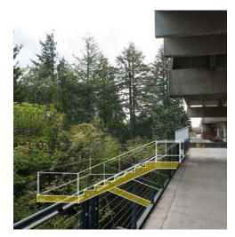
Replacement of the concrete stair tower with railings to match the existing walkway opens up views of the forest and aids wayfinding.
