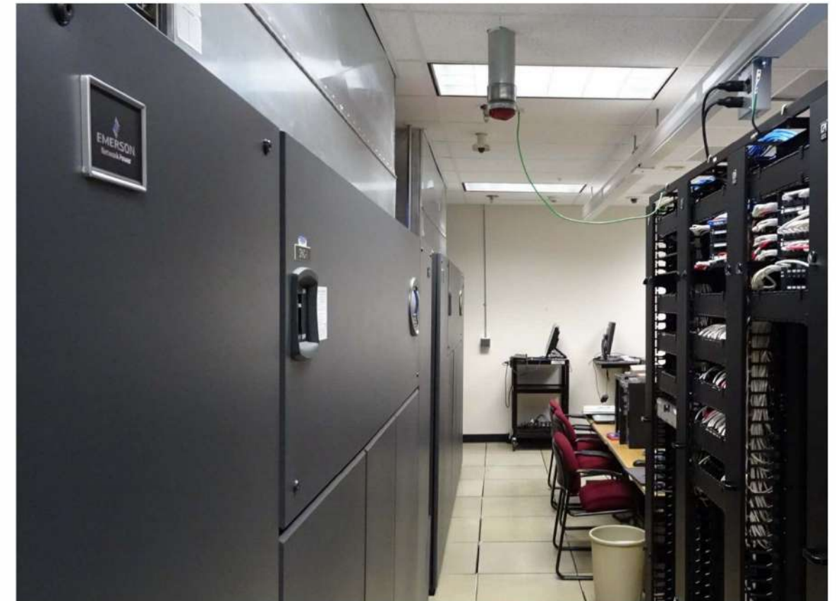
Figure 16 CRAC Units cool the hot air from the plenum above the ceiling tiles.
