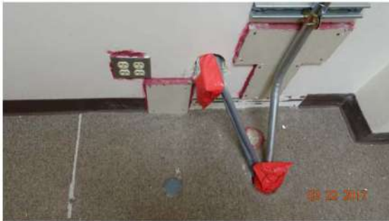
Figure 13 Poor firestopping methods.
