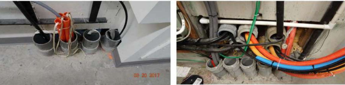
Figure 1 Example of entry conduits from other buildings.
