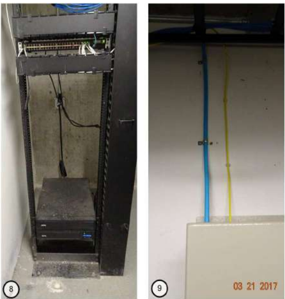
POSITIVES AND NEGATIVES OF THE IMAGES ABOVE... 8. Water, dirt from conduit directly above rack. 9. First Responder BDA COAX not sleeved through wall, no 2hr rating pathway.
