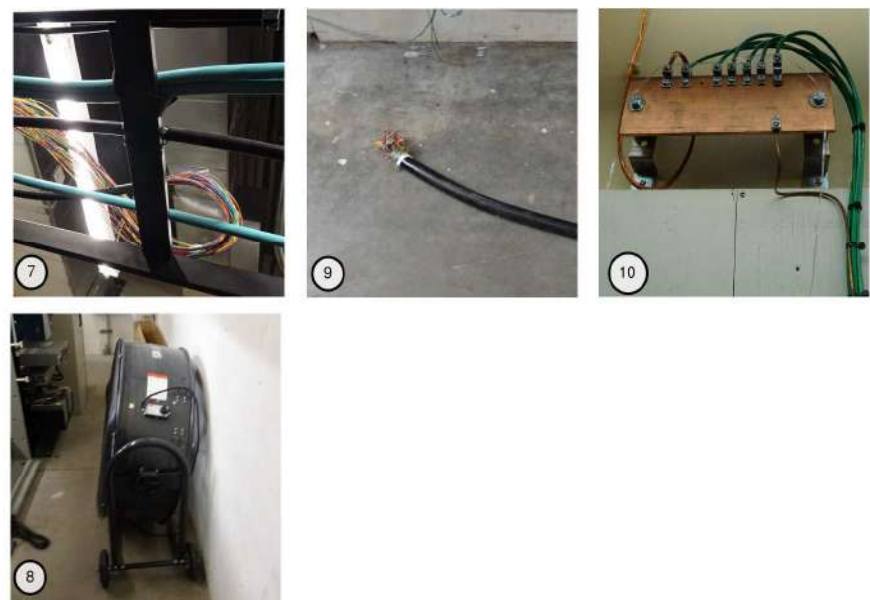
POSITIVES AND NEGATIVES OF THE IMAGES ABOVE... 7. Bare & unterminated fiber strands coiled on ladder tray – safety hazard. 8. Temporary fan in place to augment cooling. 9. Unterminated (blunt) end of copper feeder across pathway. 10. System ground conforms to PCC standard.
