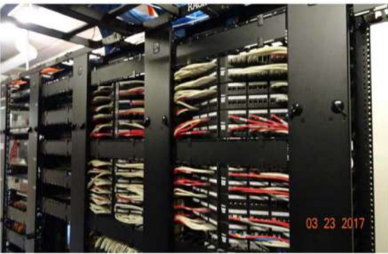
Figure 3 Example of good horizontal cable management
