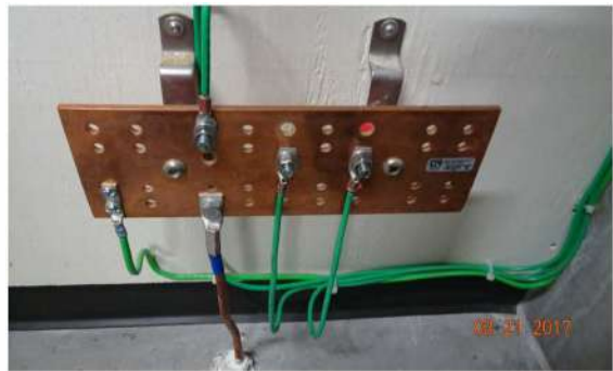
Figure 5 Example using one-hole lugs, which are no longer compliant.
