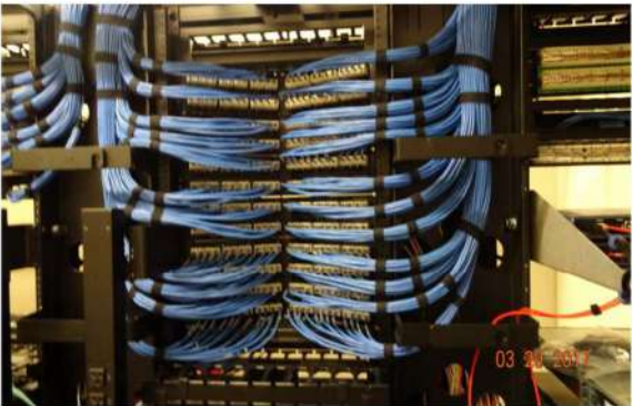
Figure 2 Terminations are well supported and easy to trace
