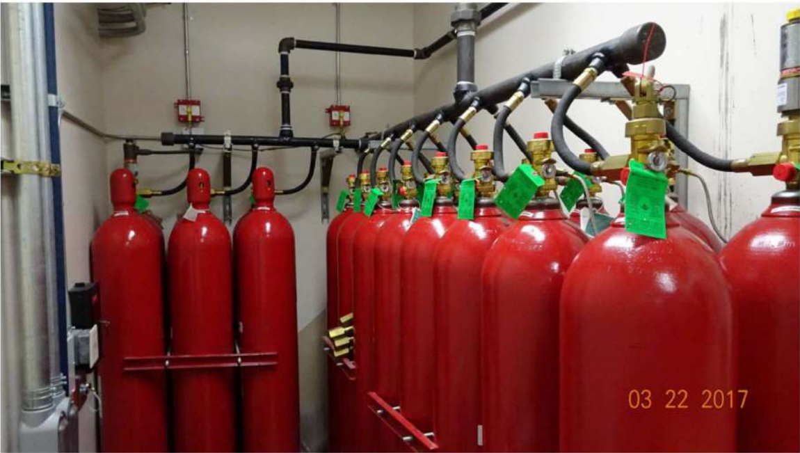
Figure 14 Inert gas suppression for data center.
