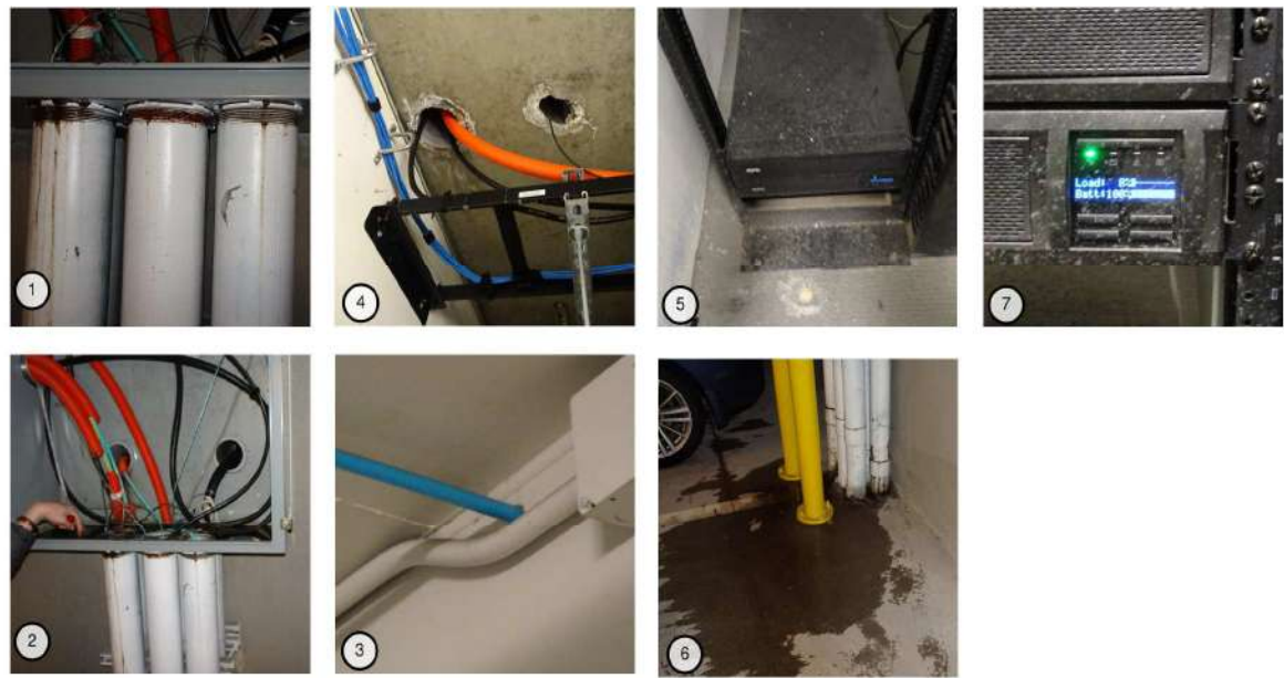
POSITIVES AND NEGATIVES OF THE IMAGES ABOVE... 1. & 2. & 6. Water infiltration of communications ducts and pull box. 3. First Responder BDA COAX not sleeved through wall, no 2hr rating pathway. 5. & 6. & 7. Water, dirt from conduit directly above rack.
