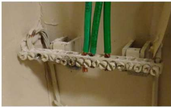
Figure 6 Ground bar is not an approved type.
