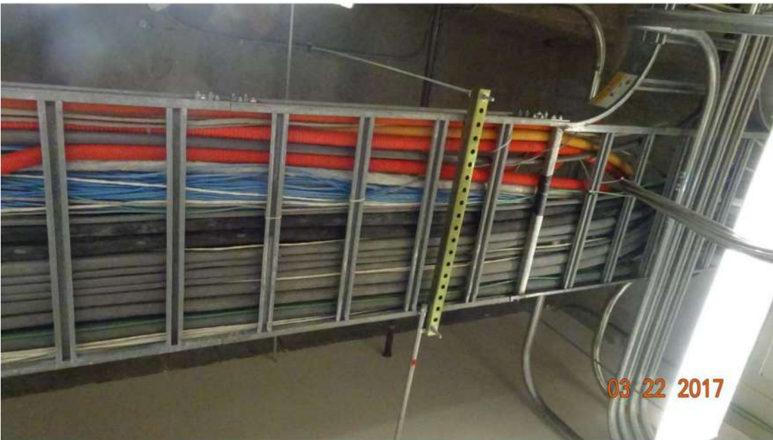
Figure 10 Overloaded tray in Sylvania tunnel system.
