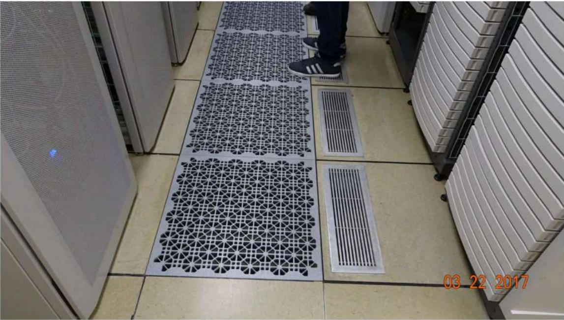
Figure 18 Cold air is directed to the aisle between cabinets, where the equipment air intakes are located.
