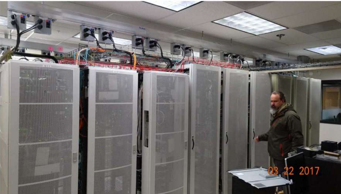
Figure 17 Rear of the cabinets face out to the room. Hot air is exhausted, rising to the ceiling return vents
