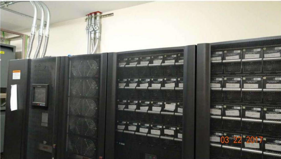
Figure 19 UPS and cabinets of batteries.
