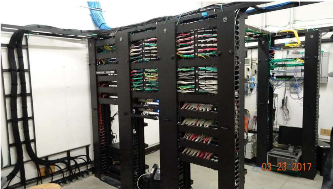
Figure 8 Good wire management, excellent capacity for expansion.
