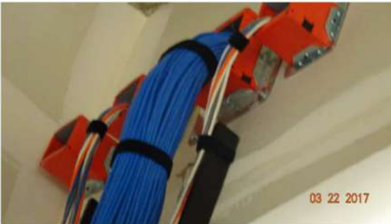
Figure 12 Good firestopping methods.
