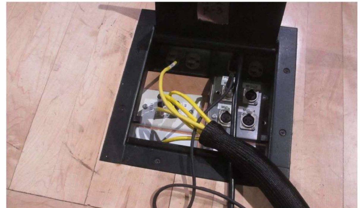
Figure 13 Stage floor connections.
