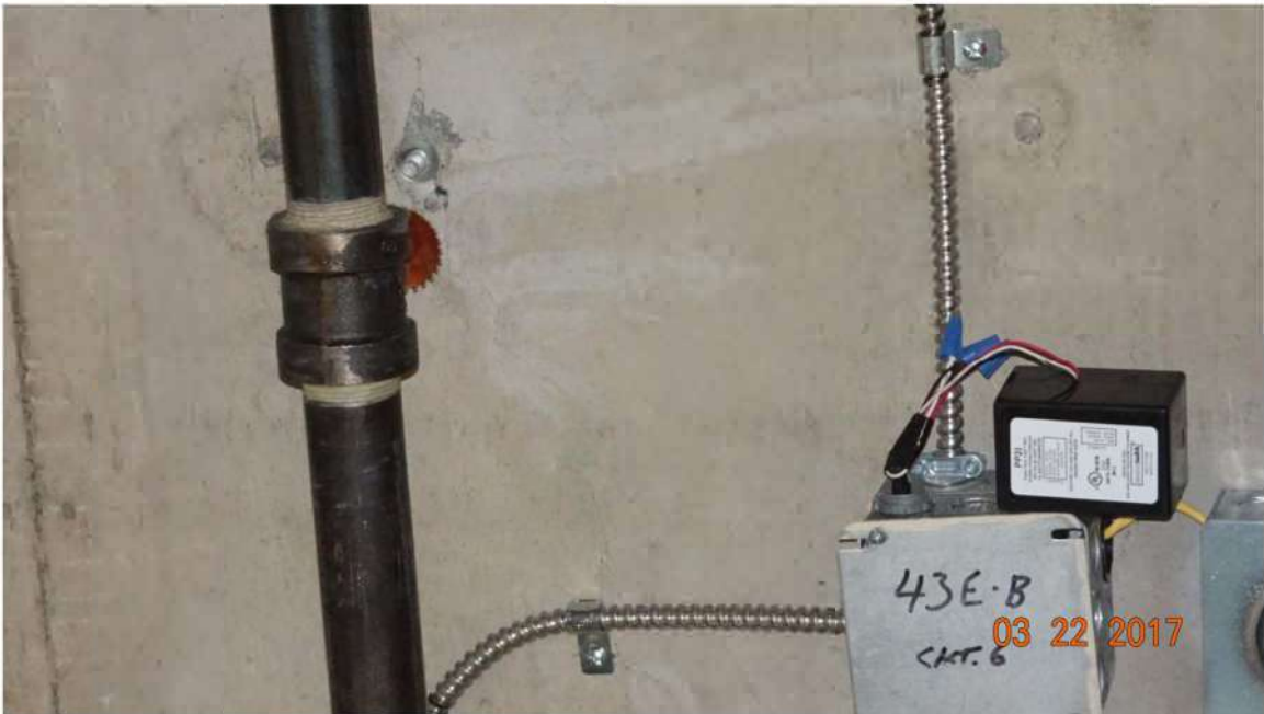
Figure 15 Sprinkler adjacent to open electrical circuits presents a hazard.
