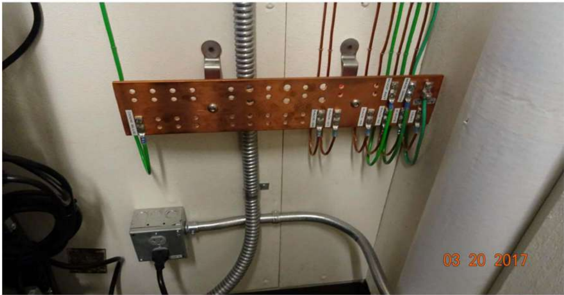
Figure 4 Example of grounding method using two-hole lugs, which comply with current standards.
