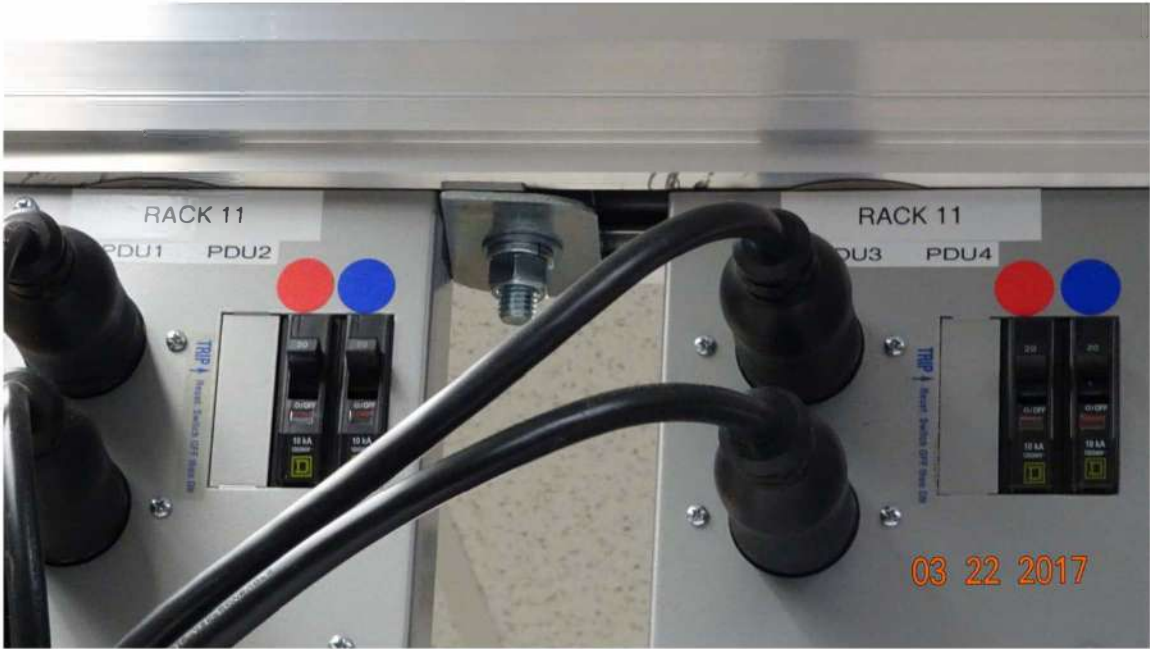
Figure 20 Starline bus with redundant circuits.
