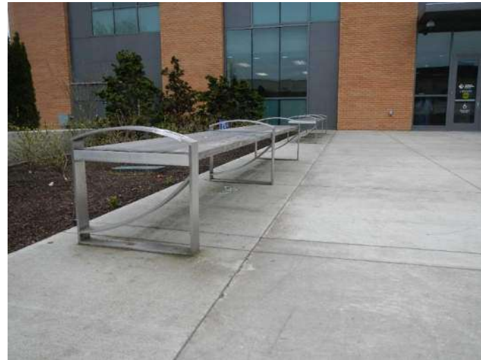
Keynote 3 Bench in front of Library with non-compliant cross slope
