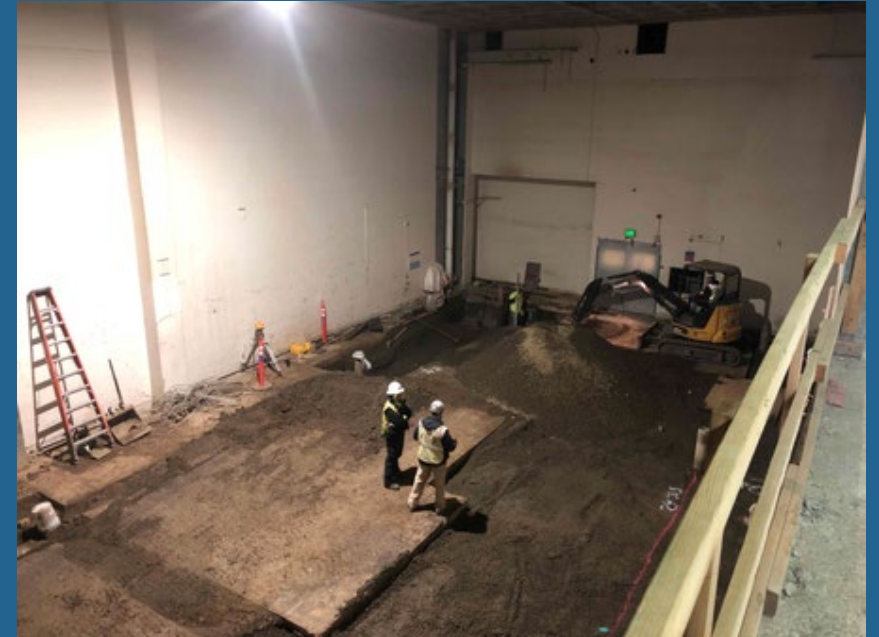
Backfilling over underground HVAC ductwork
