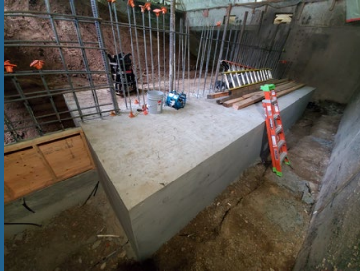
Pile cap @ GL C & 8-9 – completed last month
