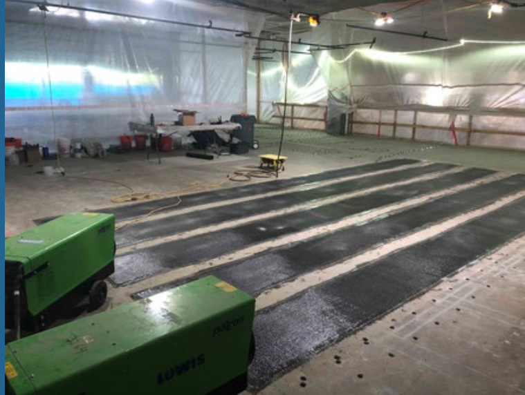
FRP install within a tempered & dust-controlled area – 2 nd floor
