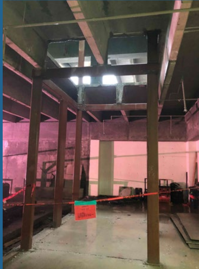
Structural Steel Framing @ Elevator shaft
