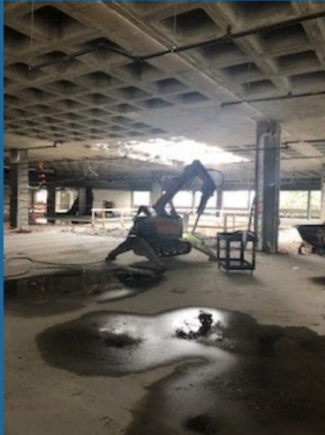
Use Brokk (a demo robot, remote control) to demo the roof opening for future HVAC duct shaft
