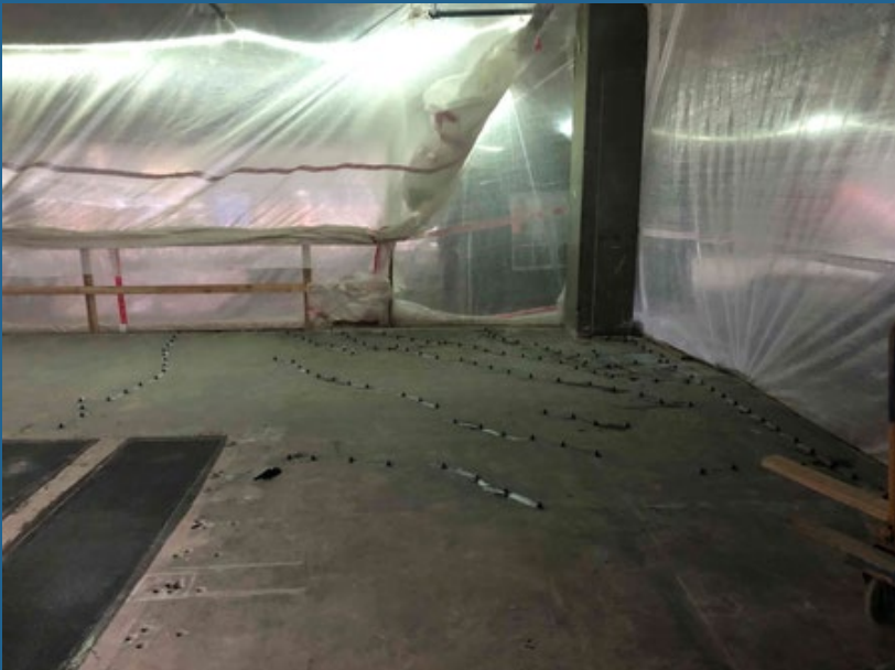
Epoxy injection @ hairline cracks on slab prior to FRP install
