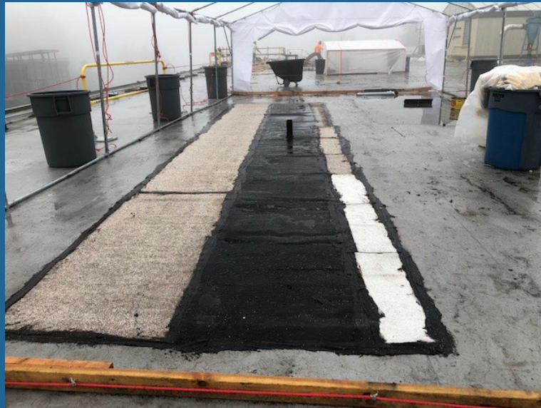
Temp roofing install over cured FRP for protection @ Roof Level
