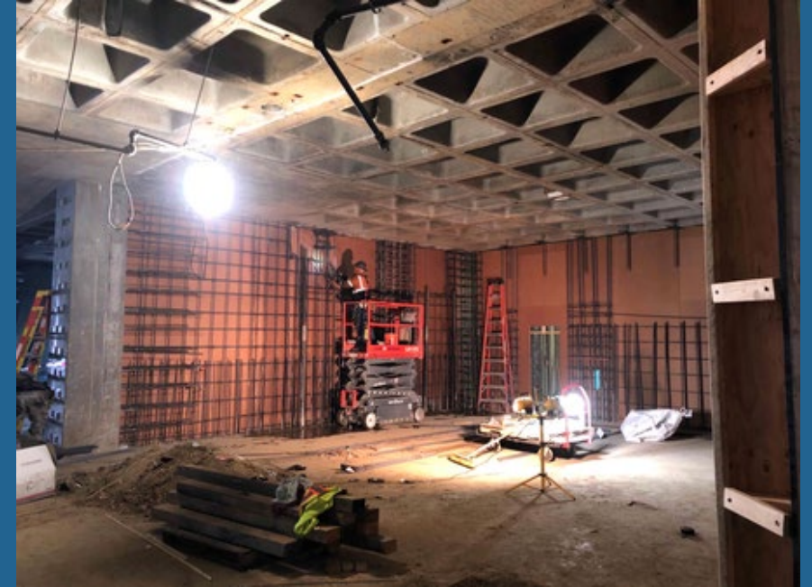
Form Shear Wall @ Mechanical Stair Shaft
