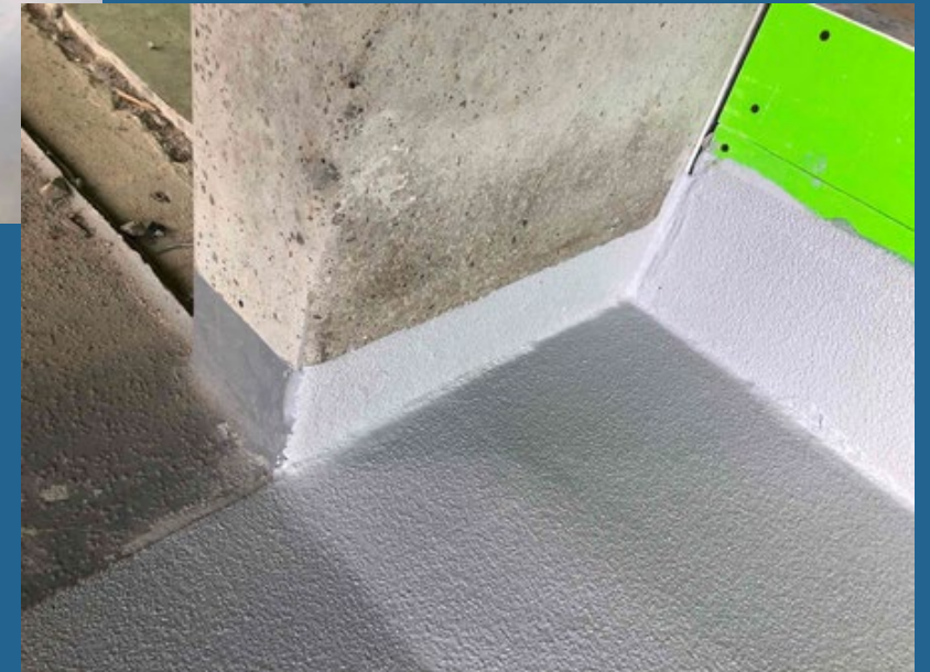
New traffic coating @ exterior mock-up
