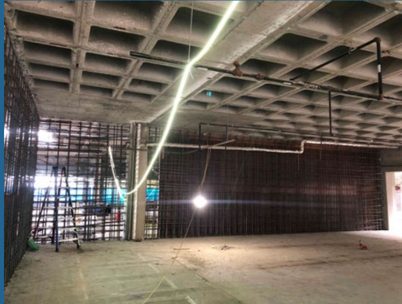
Shotcrete Shear Wall – Formwork in progress
