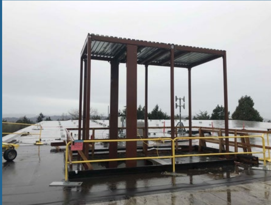
Protect elevator's opening @ roof overrun.
