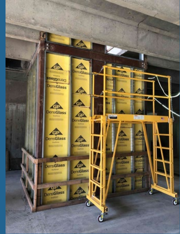
Structural steel columns at Atrium and at Elevator
