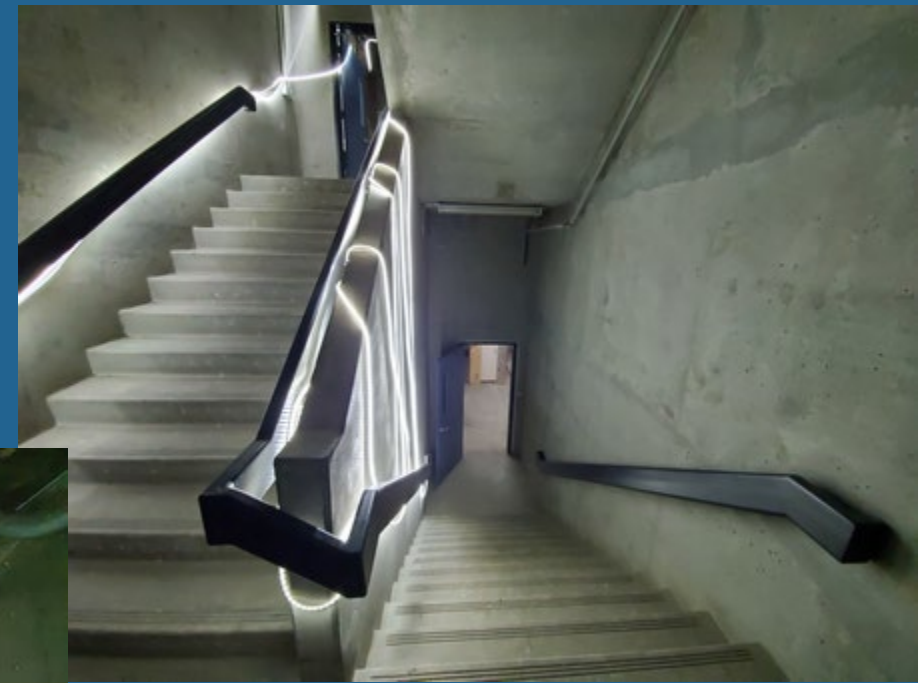
Temp lighting in stair wells
