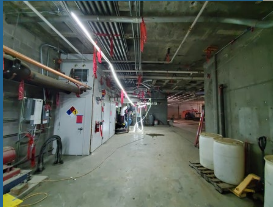
Tagged existing live power and utilities to avoid during demolition
