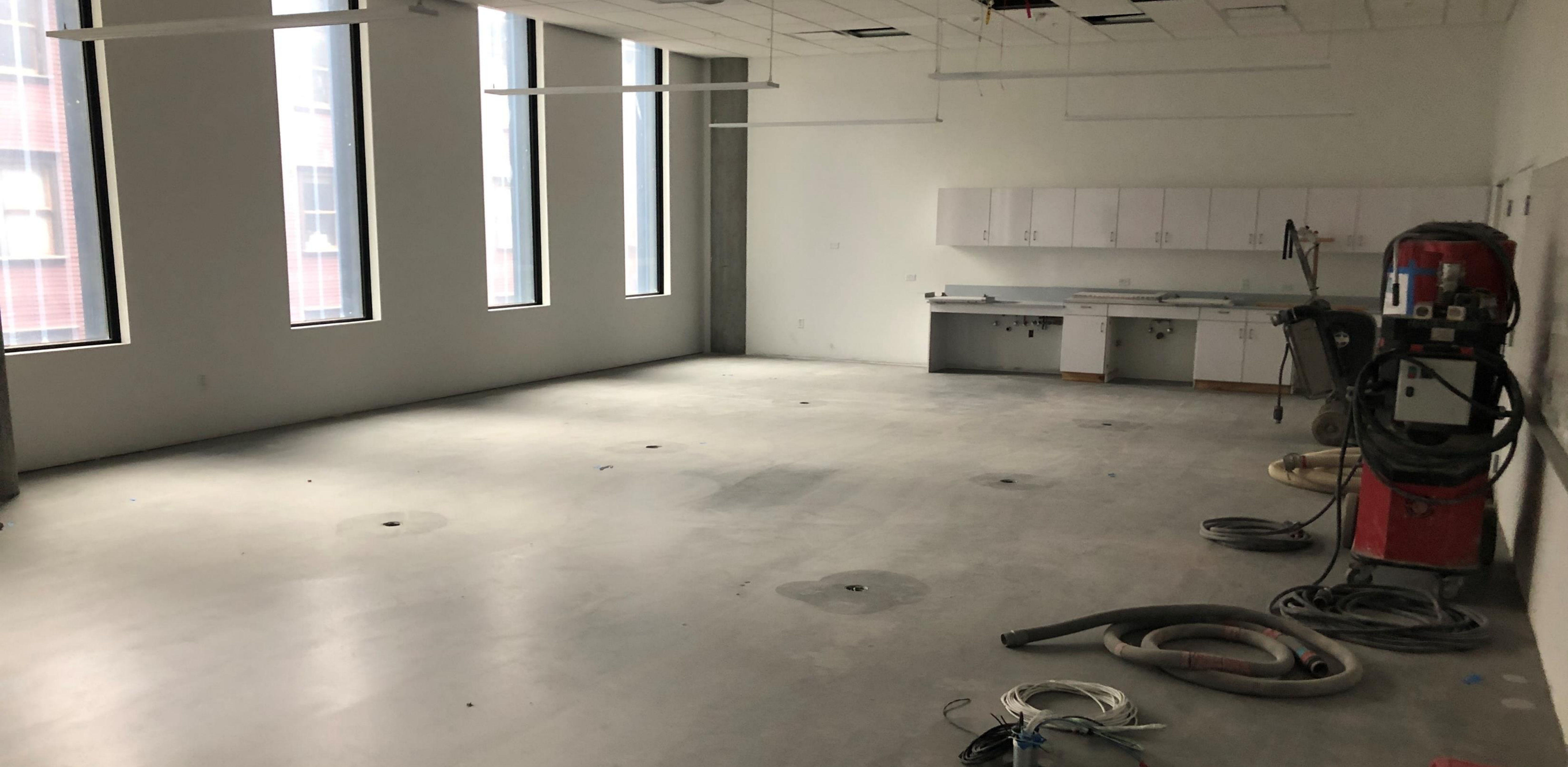
Level 2 – Stem Lab 262 Currently Polishing Concrete
