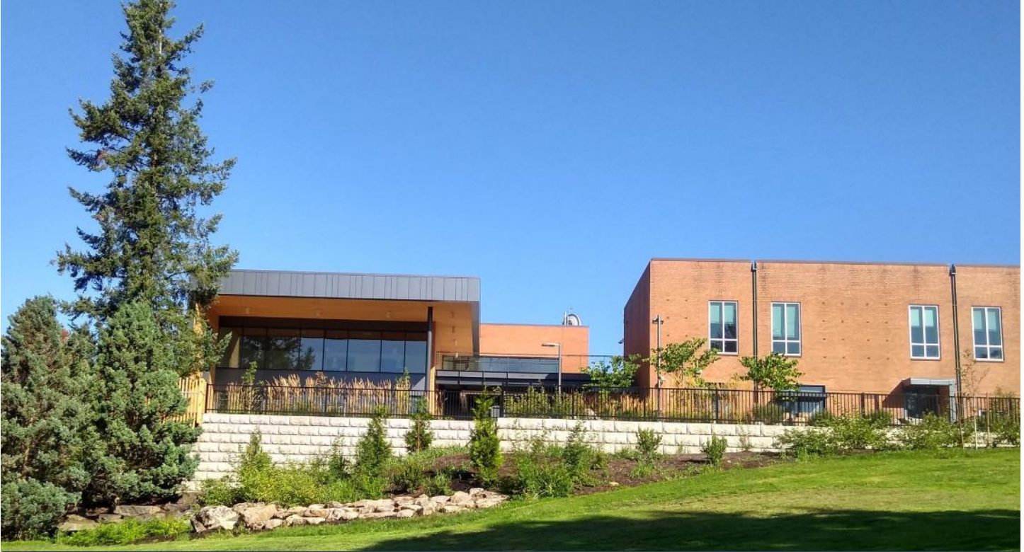
ABOVE: The new Child Development Center at Sylvania Campus
