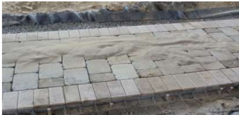
Figure 4. Sand piled on pavers.
