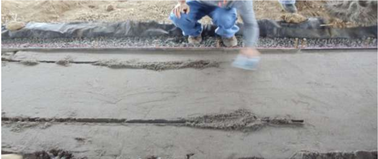
Figure 2. Finishing the sand bed.
