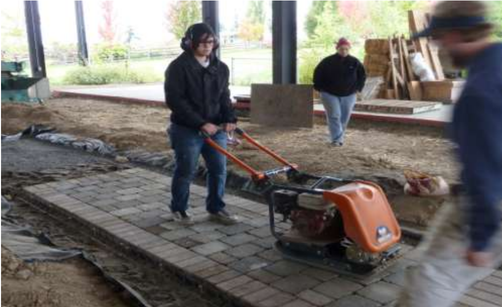
Figure 5. Finishing with the plate compactor.
