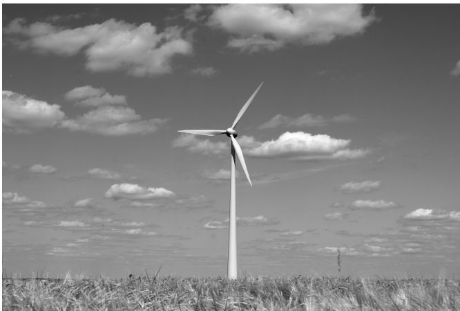
Rural wind turbine
